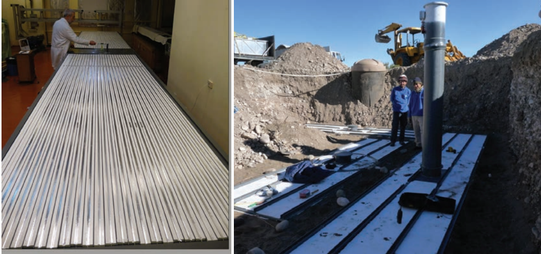
Figure 11. (Left) A 10 m 2 module being assembled and (Right) its deployment at the Observatory site.
